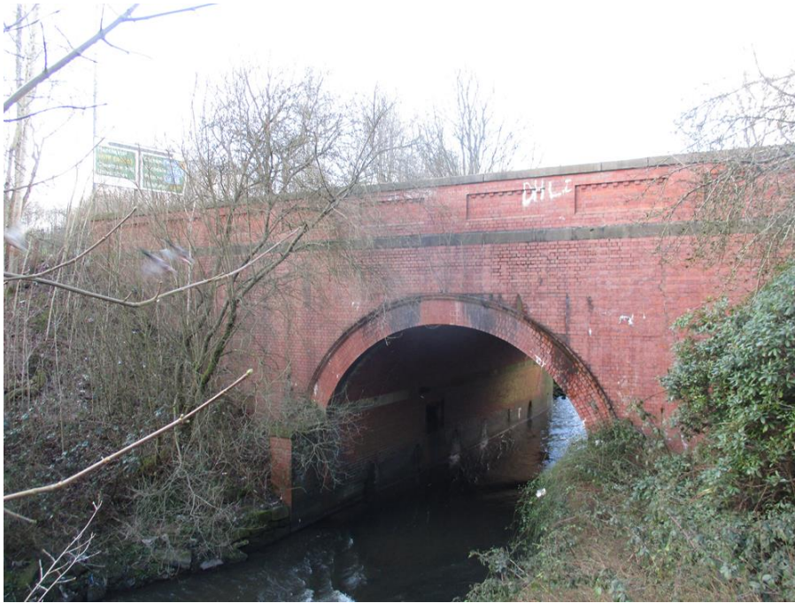
Victoria Avenue Bridge (River Irk)
