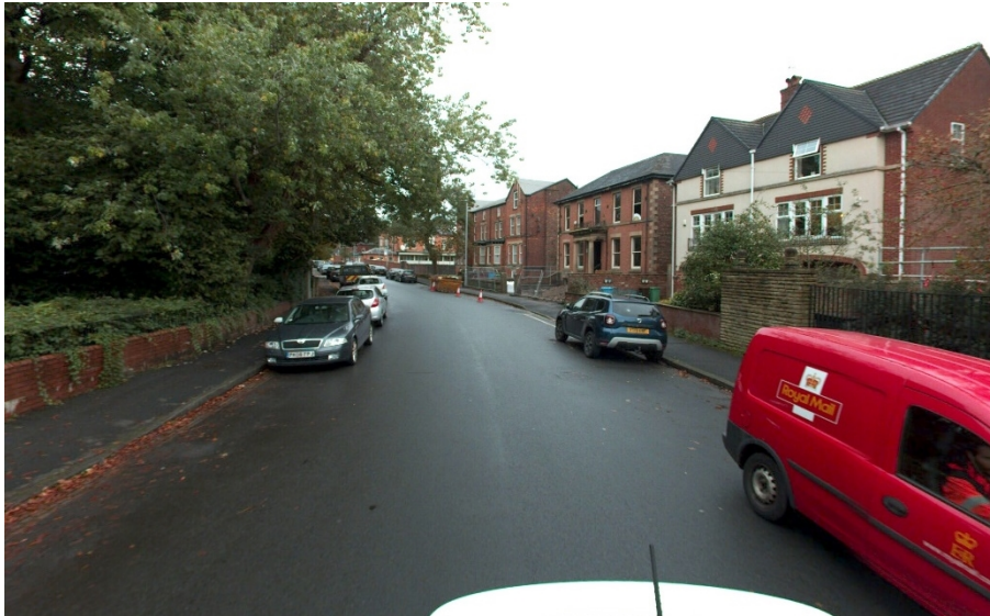
Manchester Road, Chorlton – before and after resurfacing works.
